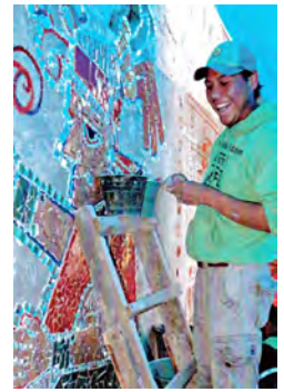
Cementing the tiles
