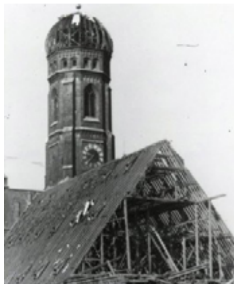
Munich Frauenkirche "dome" with wooden beams exposed, circa 1945.
