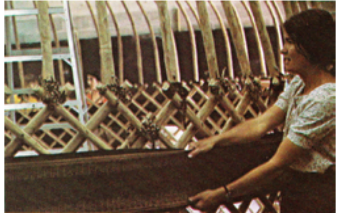
Handwoven bands are tightened around the perimeter of the yurt's lattice framework by Ann Bliss.
