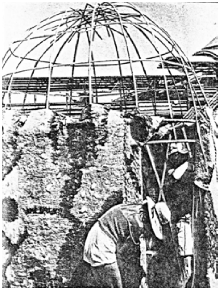
Hey Frey and John Guest stitch felted panels to the yurt's lattice structure.
